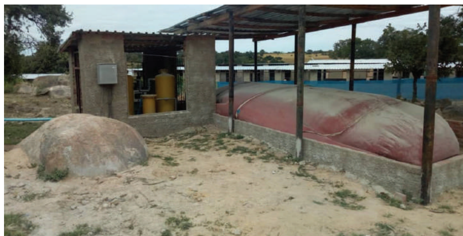
Biogas digester, generator tank
